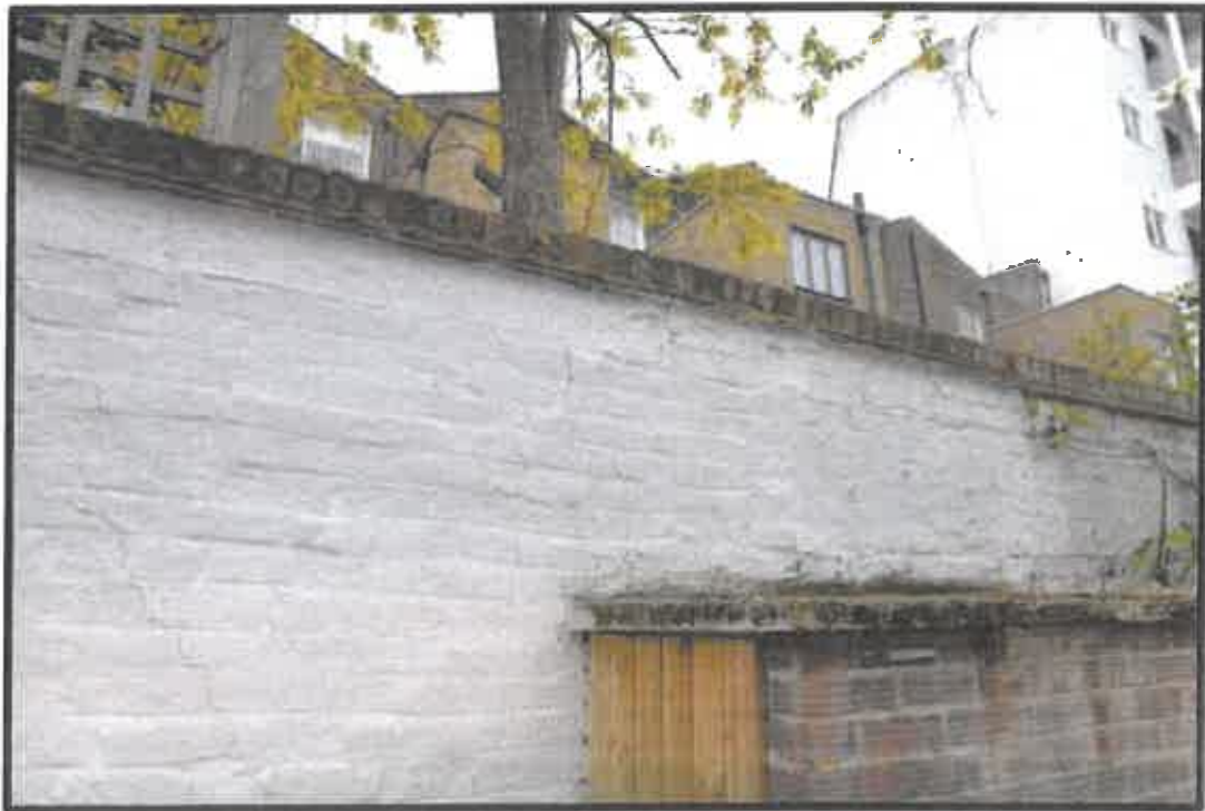
Picture showing the extensive cracking of the boundary wall.
